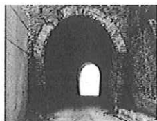
Uscita tunnel Via Respighi
